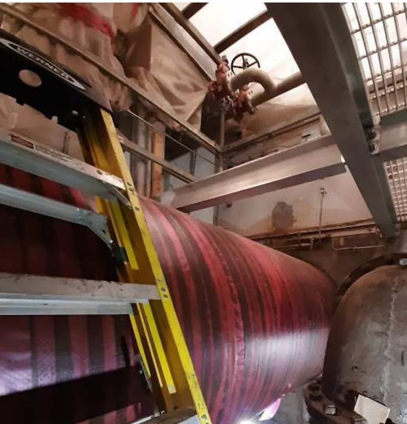
Customer received an ISO/ASME compliant repair system able to stop the corrosion, return the mechanical strength back to the water pipe and designed to provide a 20 year lifetime.
